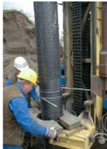
installation of push fit/spring lock coupling
