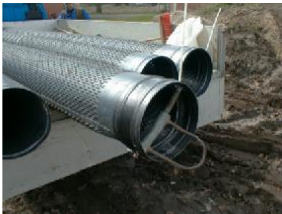
bridge slotted screens for dewatering purposes with lifting cap
