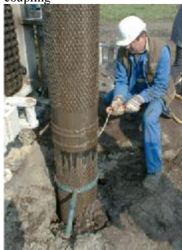
dismantling of retrieved assembly
